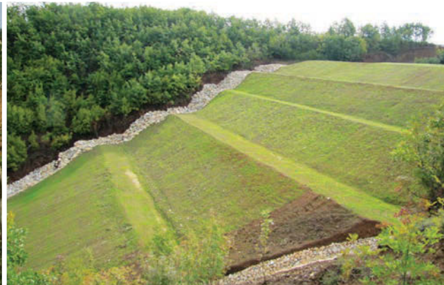
Figure 9 → Reshaped dam from and water diversion channels installed left and right of the dam wall
