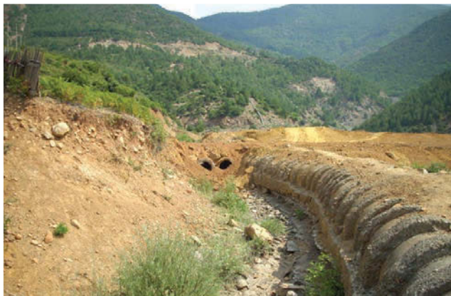
Figure 6 → Reconstructed water diversion channel
