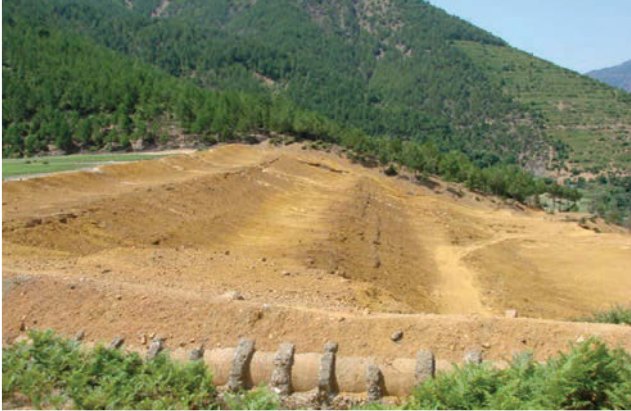
Figure 5 → Stabilized dam face
