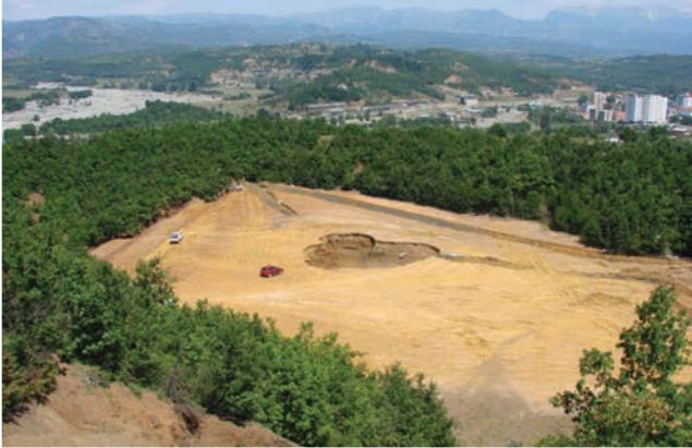
Figure 8 → Sinkhole removed and dam surface covered
