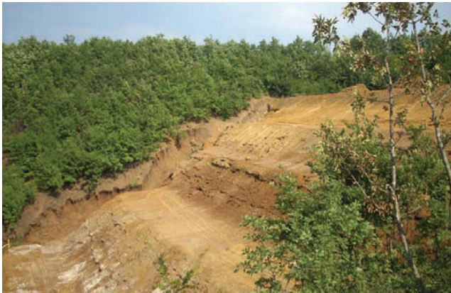
Figure 9 → Reshaped dam from and water diversion channels installed left and right of the dam wall
