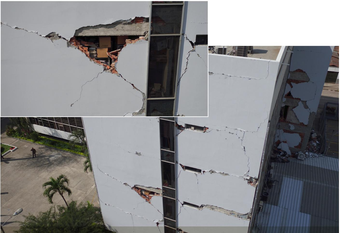
**Figure 4** An earthquake-damaged building from a bird’s eye view, taken by the Phantom 1 pro. Here it’s possible to show the extent of damage and to provide an educated estimate on the safety of a structure. AeroVison, May 2016.
