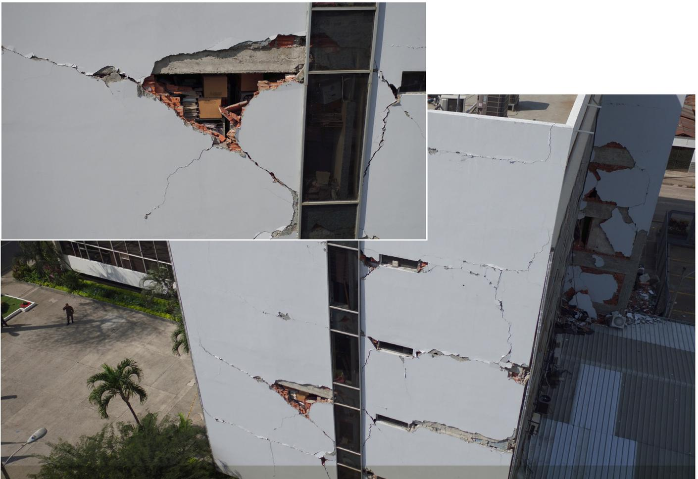
**Figure 4** An earthquake-damaged building from a bird’s eye view, taken by the Phantom 1 pro. Here it’s possible to show the extent of damage and to provide an educated estimate on the safety of a structure. AeroVision, May 2016.
