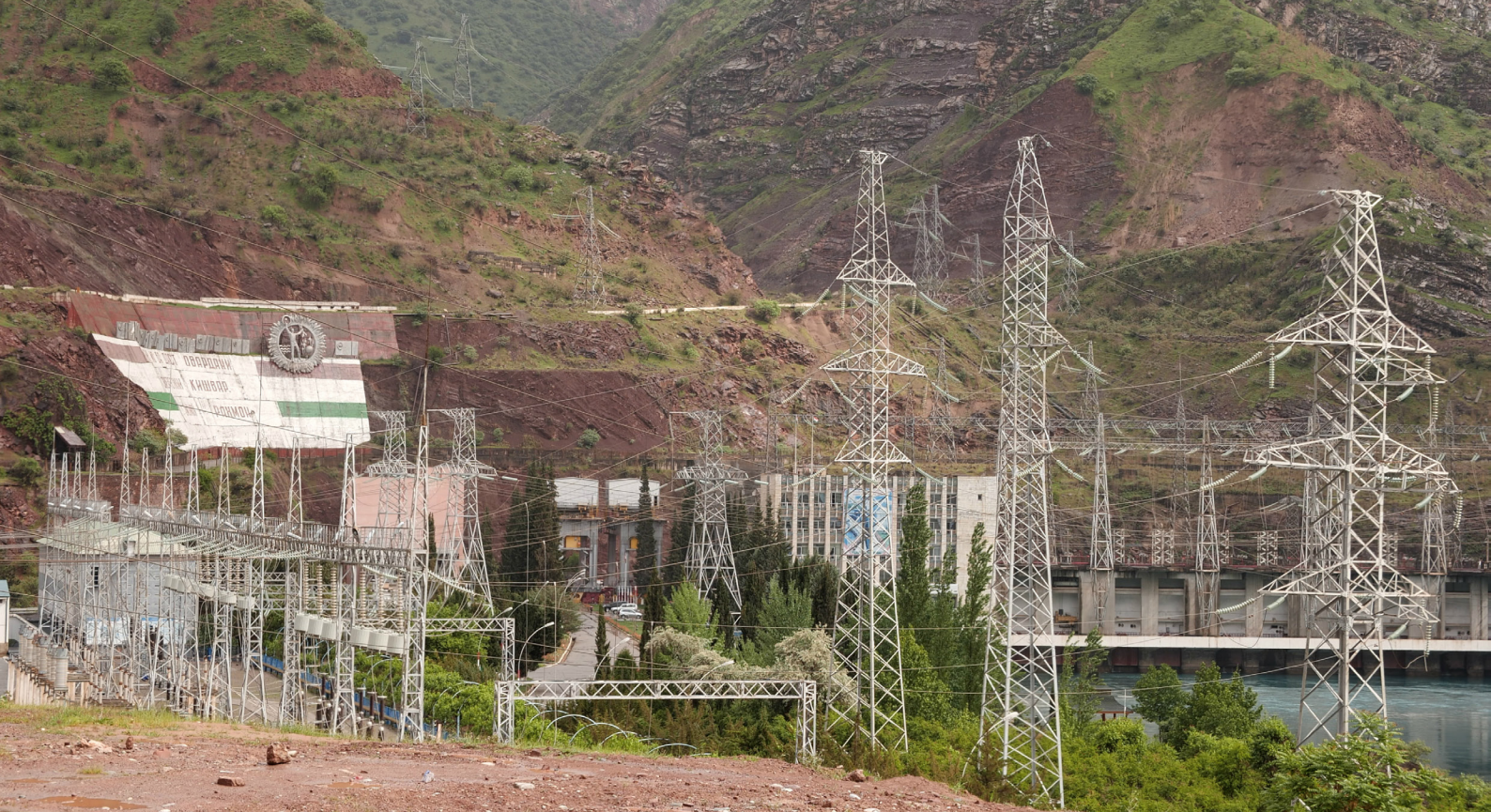
© Zoï Environment Network / Christina Stuhlberger Nurek hydropower station and infrastructure, Tajikistan
