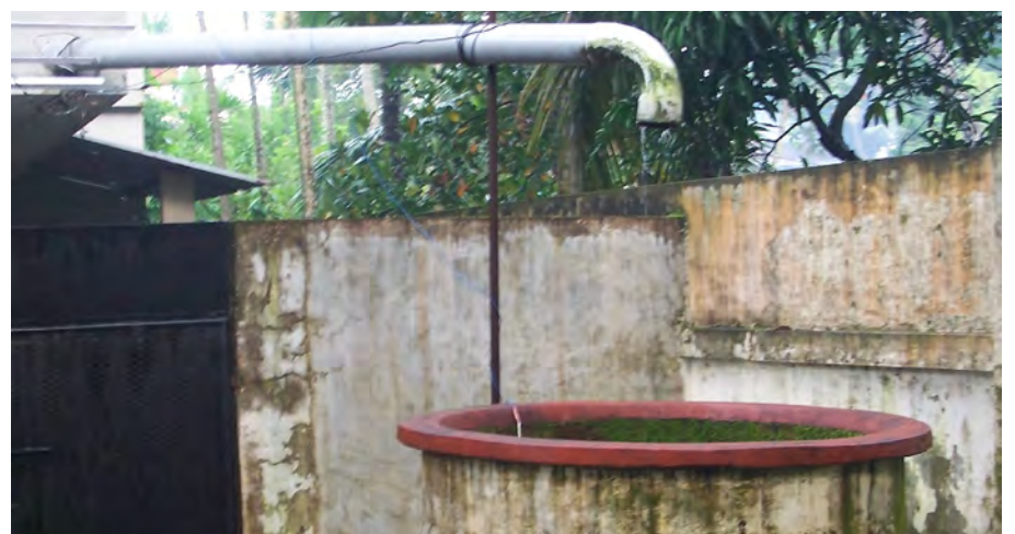
PVC structure with elevated well wall to prevent overflow. KC Bellarmine.
