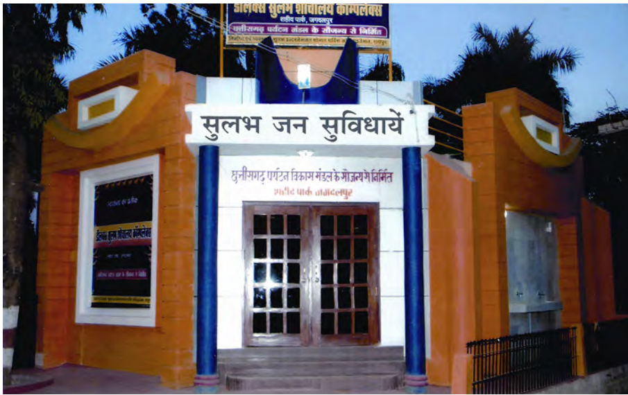
Sulabh's coin operated toilet facilities provide low cost sanitation to poor consumers. Sulabh.
