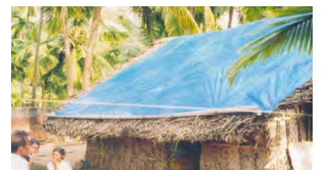
Masonry work to collect rain water on a tiled roof. Planet Kerala.
