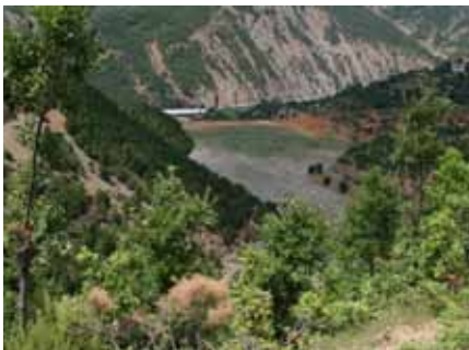
View on Reps tailings dam
