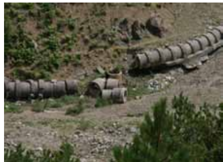
Failed water diversion channel
