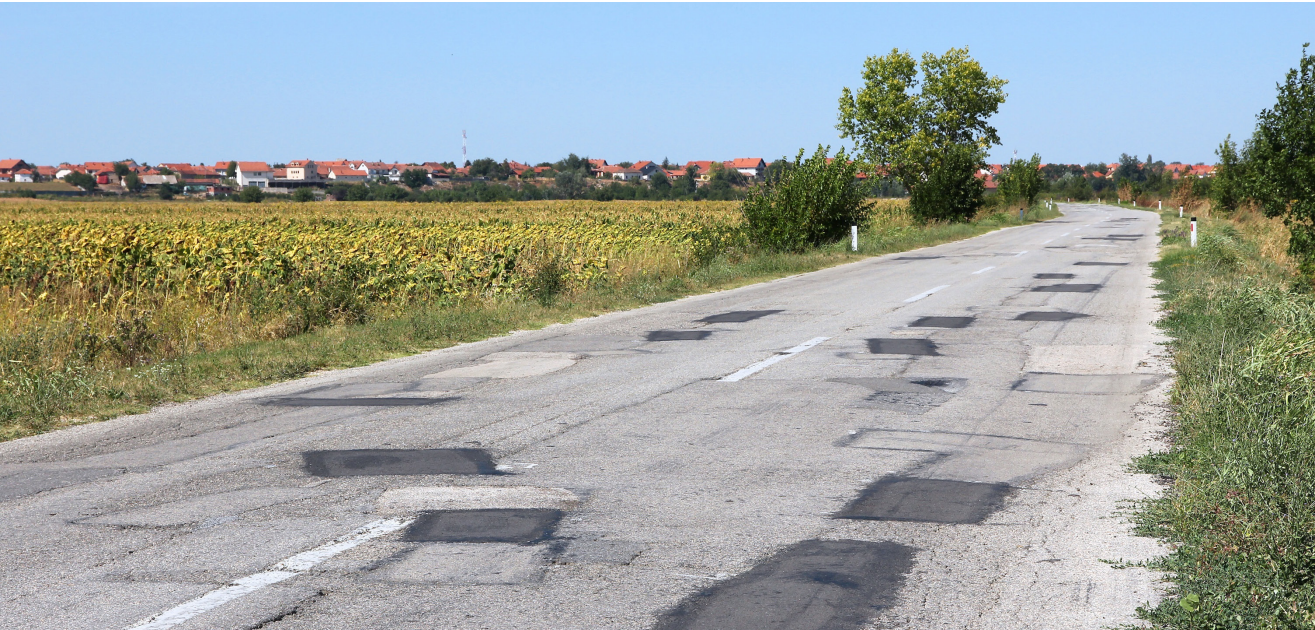
Poorly patched road in Negotin, Serbia. Regional road in Bor district of Serbia.
