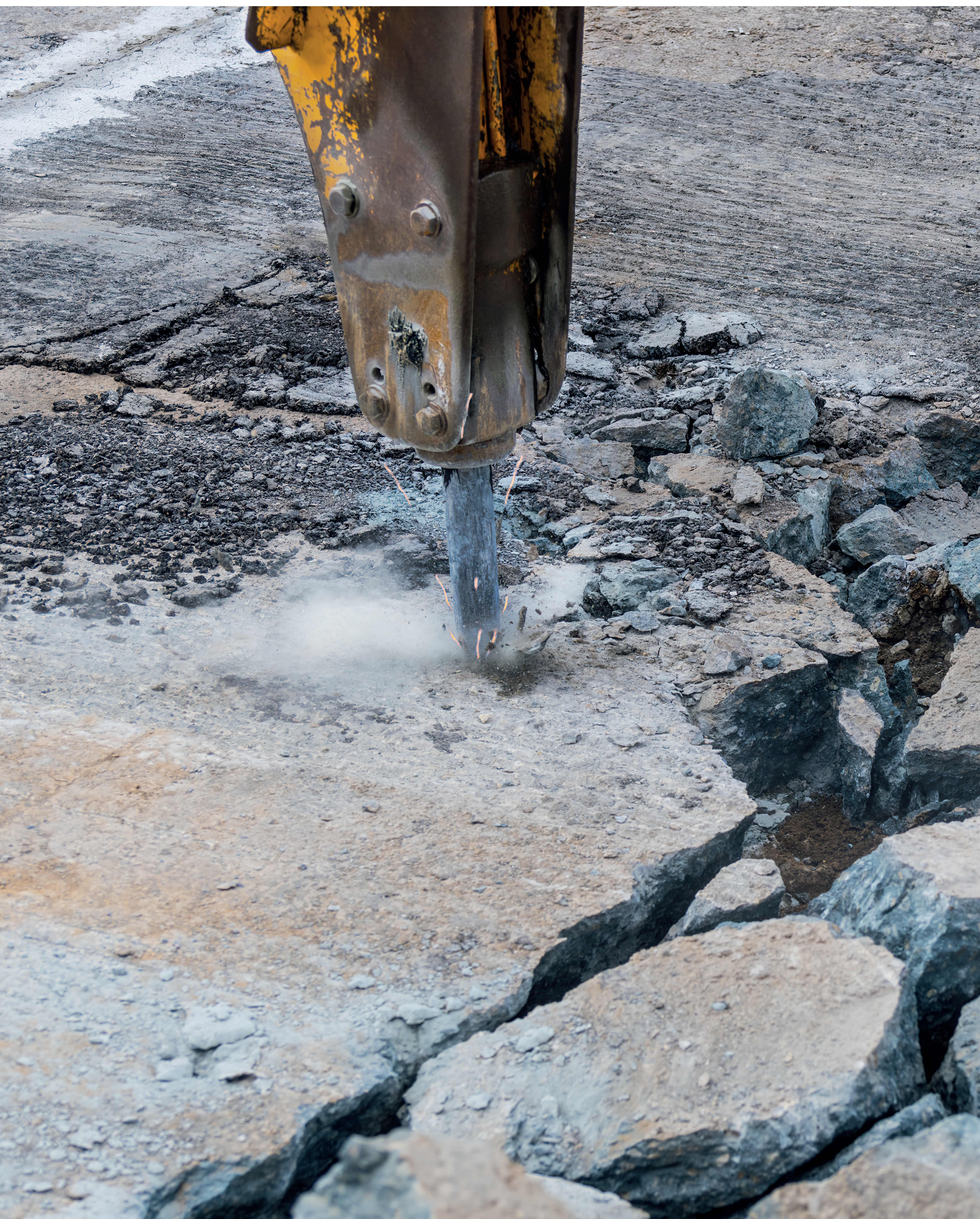
Demolition hammer and broken concrete pieces.
